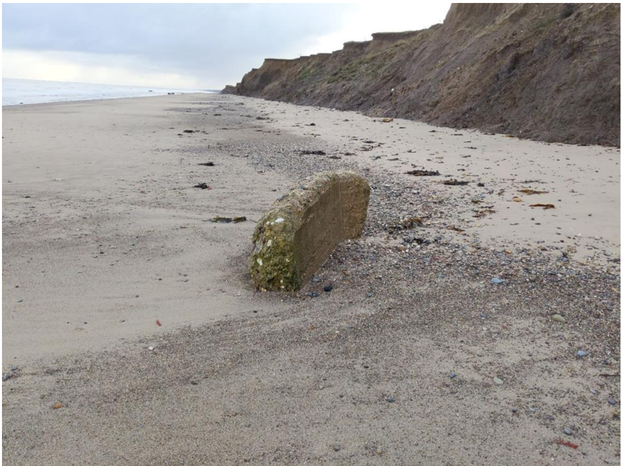
Plate 22-4-3 View of concrete remains of WWII pillbox remains (21233)
